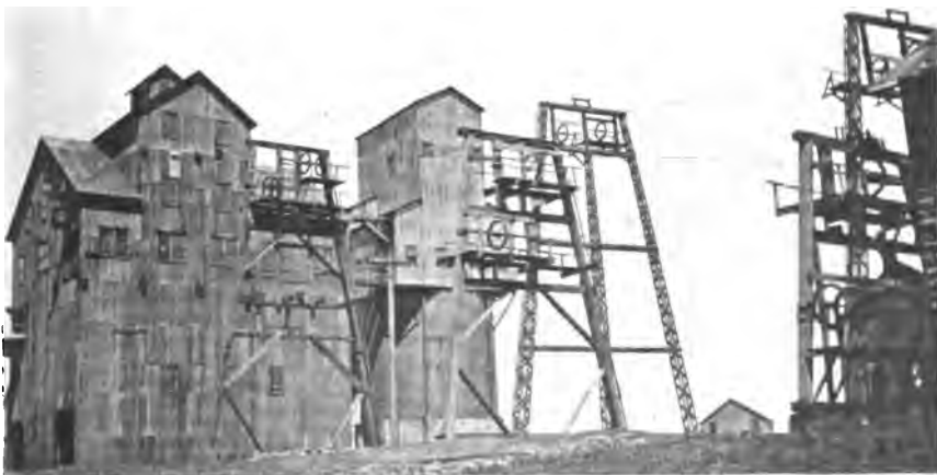
B. ROCK HOUSES, OLD AND NEW TYPES, CENTENNIAL MINE.
